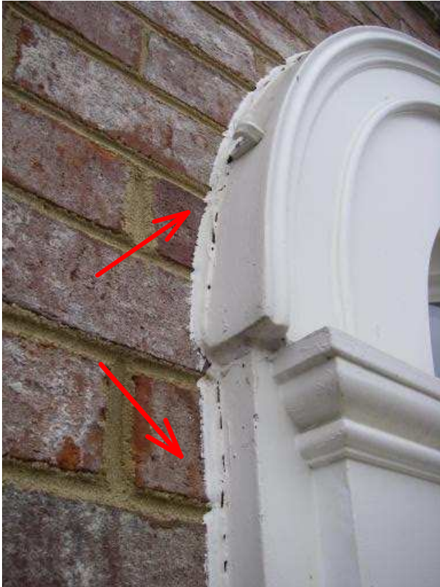
Caulk and seal exterior trims where needed
