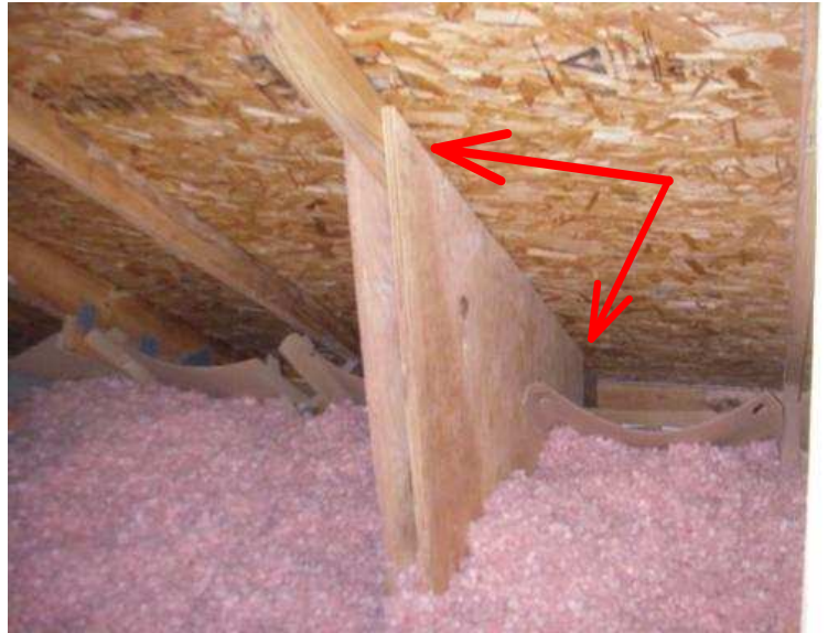
Modified roof truss
